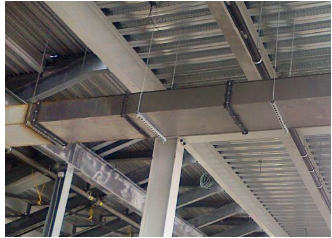
DuraDuct™ SED connected to existing exhaust system.
